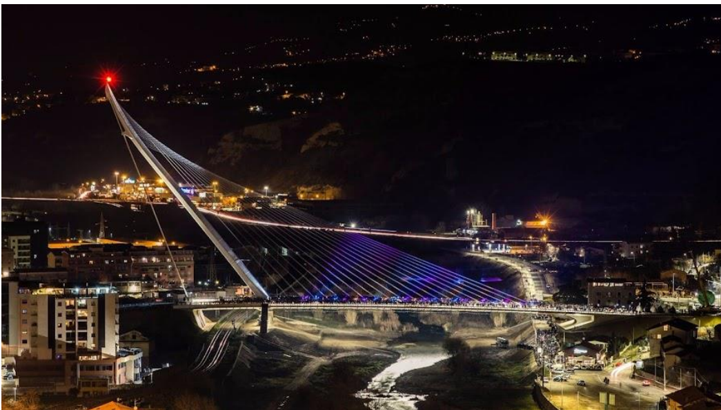
Calatrava Bridge inauguration
